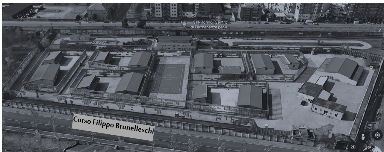
Figure 11- View of the CPR in Turin. Picture from Google earth in June 2023 (3)
