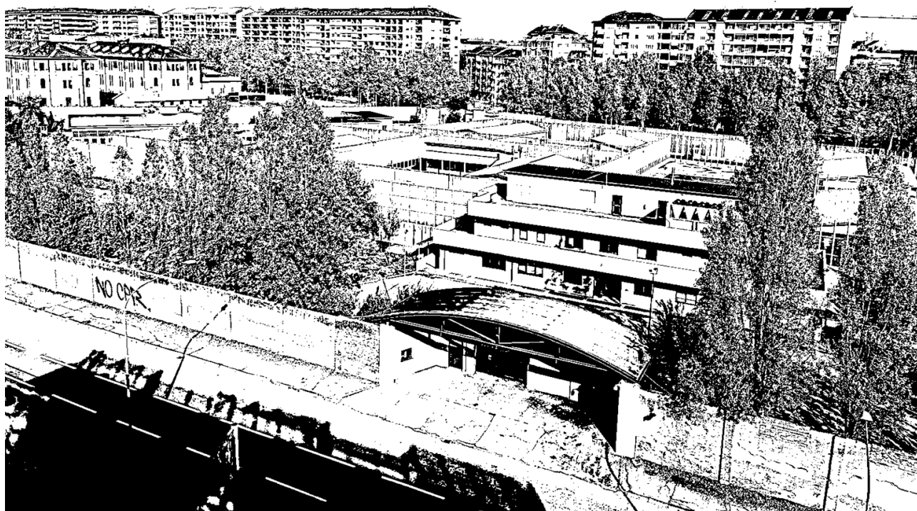
Figure 1- Picture of the view over the CPR taken from a construction scaffolding (Turin, October 2024)
