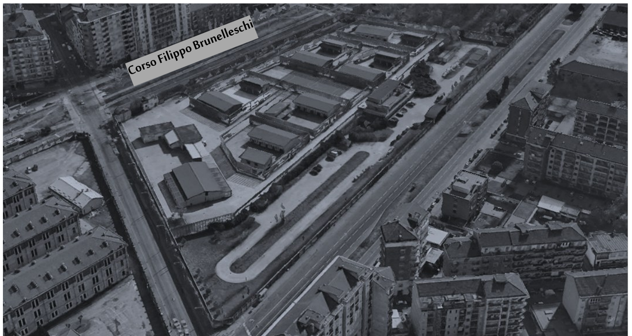
Figure 70 - View of the CPR in Turin. Picture from Google earth in June 2023 (2)
