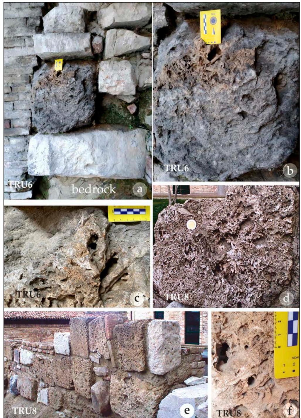
Figure 2. Remnants of defensive Roman walls which are present in the historical centre of the city (a–f). Places are located in Figure 1 and reported in Table 1 according to the label numbers (TRU). The wall reported in (e) at Palazzo Battiferri, is no longer visible due to renovations of the garden.
