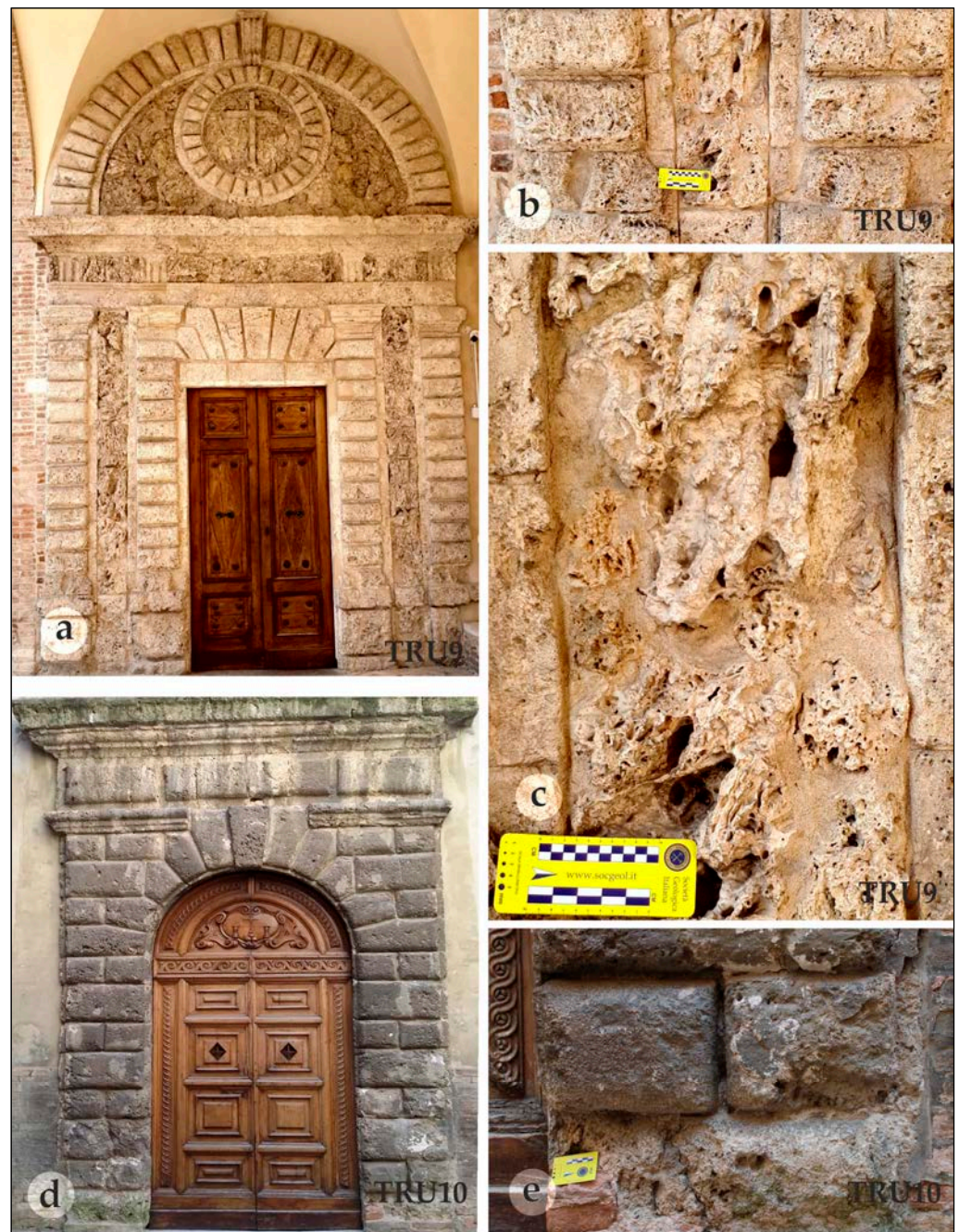
Figure 4. The two important portals of the Oratorio delle Grotte (a–c) and Oratorio della Morte (d,e) where the calcareous tufas were employed as ornamental stone. Places are located in Figure 1 and reported in Table 1 according to the label numbers (TRU).
