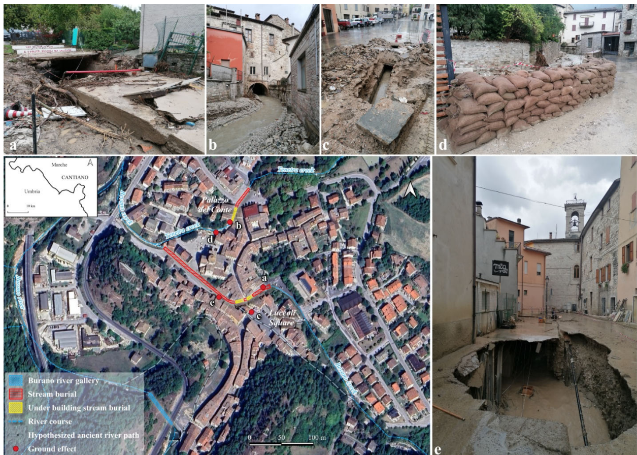
Fig. 4 Location of the effects of the high flow rates in the artificial stretch of riverbeds and sewer system within the built-up area of Cantiano. (a) pavement and road torn off by the overflowing water of the Bevano creek; (b) outlet of the underground riverbed of the Tenetra stream and related material transported; (c) break in the sewerage network in front of the Municipality; (d) natural protections set up during the emergency; (e) breaking point of the culvert caused by the high hydraulic pressure created.
