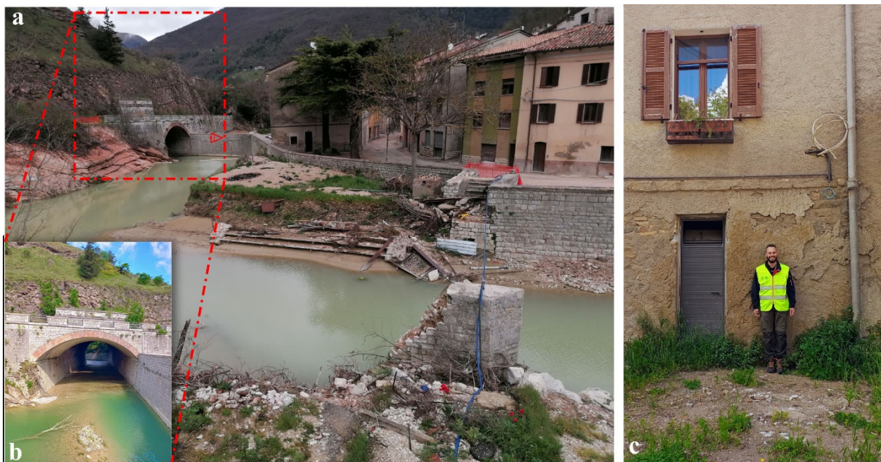
Fig. 5 (a) River stretch before the detour, flood damage can be seen; below is a destroyed bridge; (b) Burano detour tunnel as seen from the road; (c) hydrometric level reached homes near the detour area.
