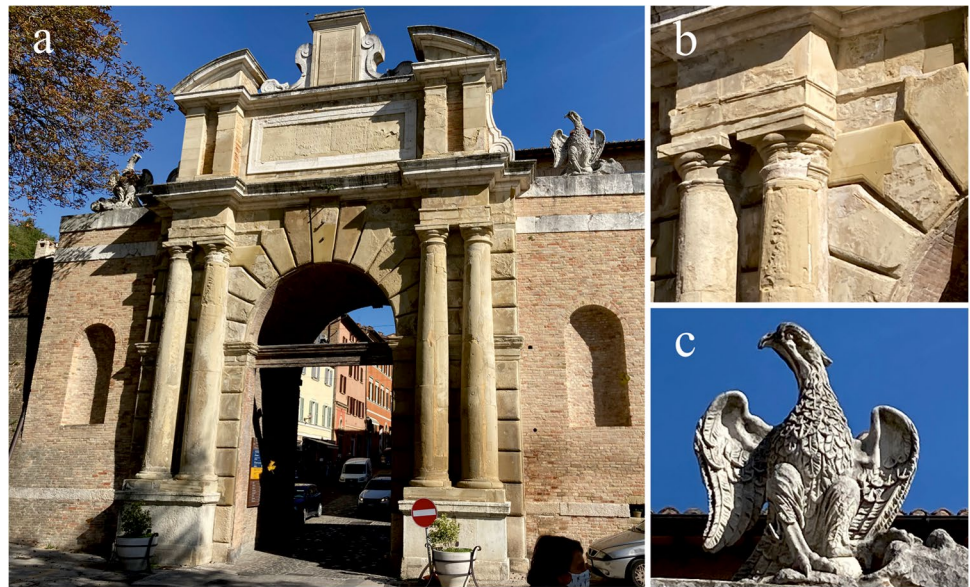
Fig. 13 Stop 10: the Porta Valbona , South-Western entrance of the historic centre of Urbino, made of the Sant’ Ippolito sandstones (a, b); detail of one of the two eagles sculpted in Calcare Massiccio Formation (c)
