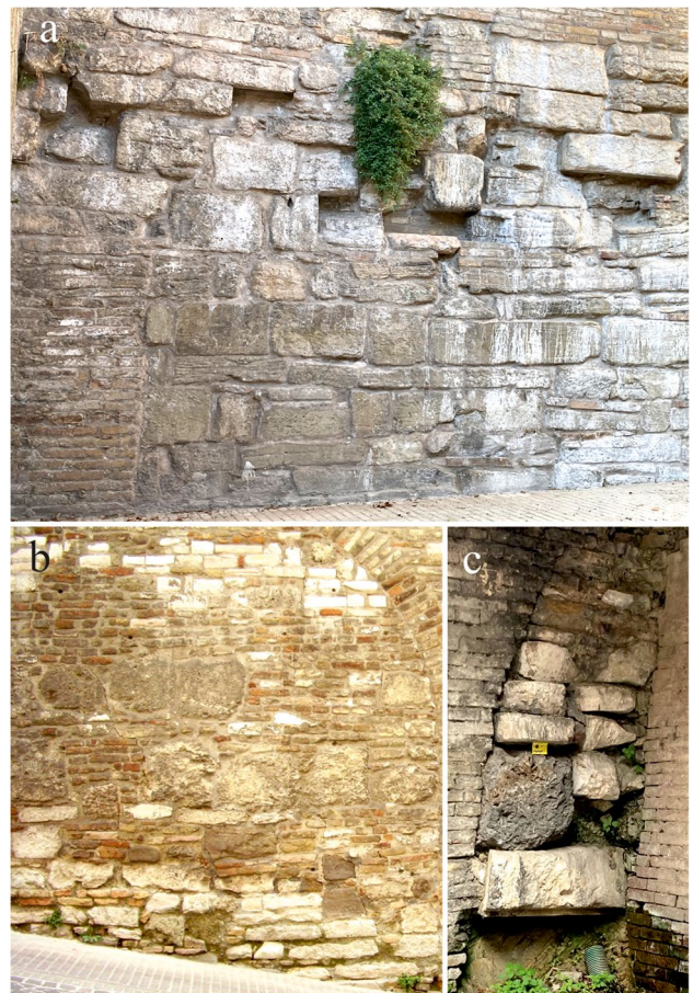
Fig. 7 Stop 5: the unique exposed remnants of the Roman walls (via Budassi ) constituted by big ashlars of travertine, nodular limestone and sandstone (a), and more recent urban fabric, via Saffi (b) and Corso Garibaldi (c), also indicated in Fig. 2 (circled letters a and b respectively) where reused Roman ashlars are present
